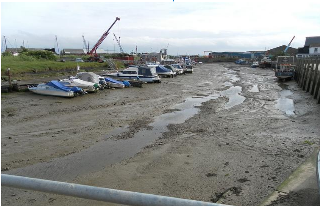
With the water not impounded
